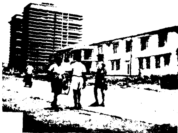
THE AFRICAN CONTINENTAL BANK. This fine tall building was recently completed at Enugu, Nigeria.
