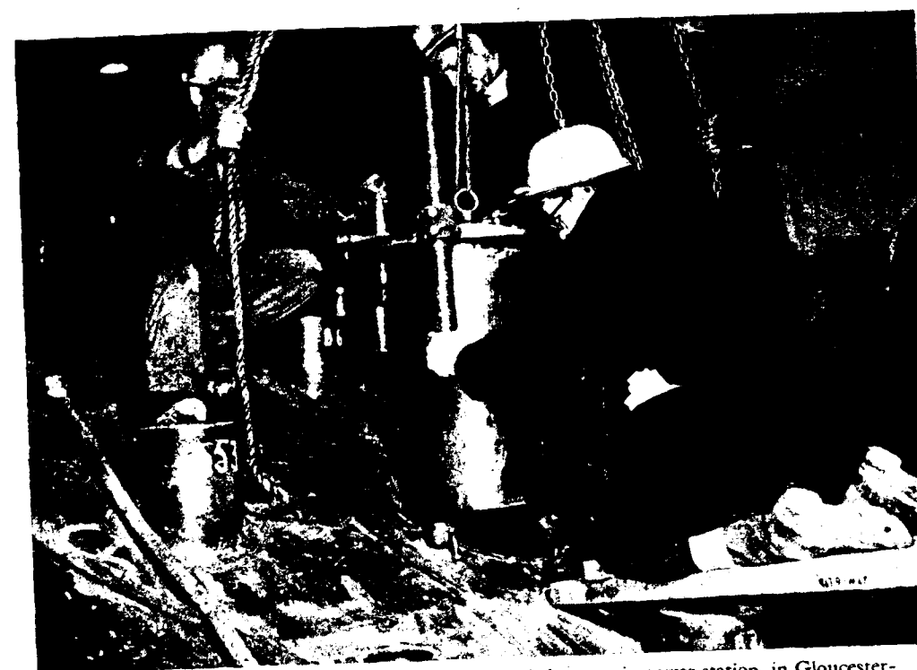
WELDERS at work inside No. 1 reactor vessel at the Berkeley atomic power station, in Gloucestershire, the first commercial nuclear power station to be started in Britain. Below: The Fast Fission Breeder Reactor set up by the U.K. Atomic Energy Authority at Dounreay, Caithness, Scotland.
