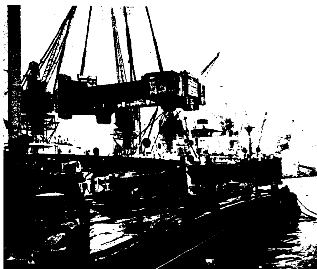
MILL MACHINERY for Durgapur. The first of two 74-ton roll housings manufactured by a Sheffield engineering firm is swung aboard ship at Birkenhead docks.
