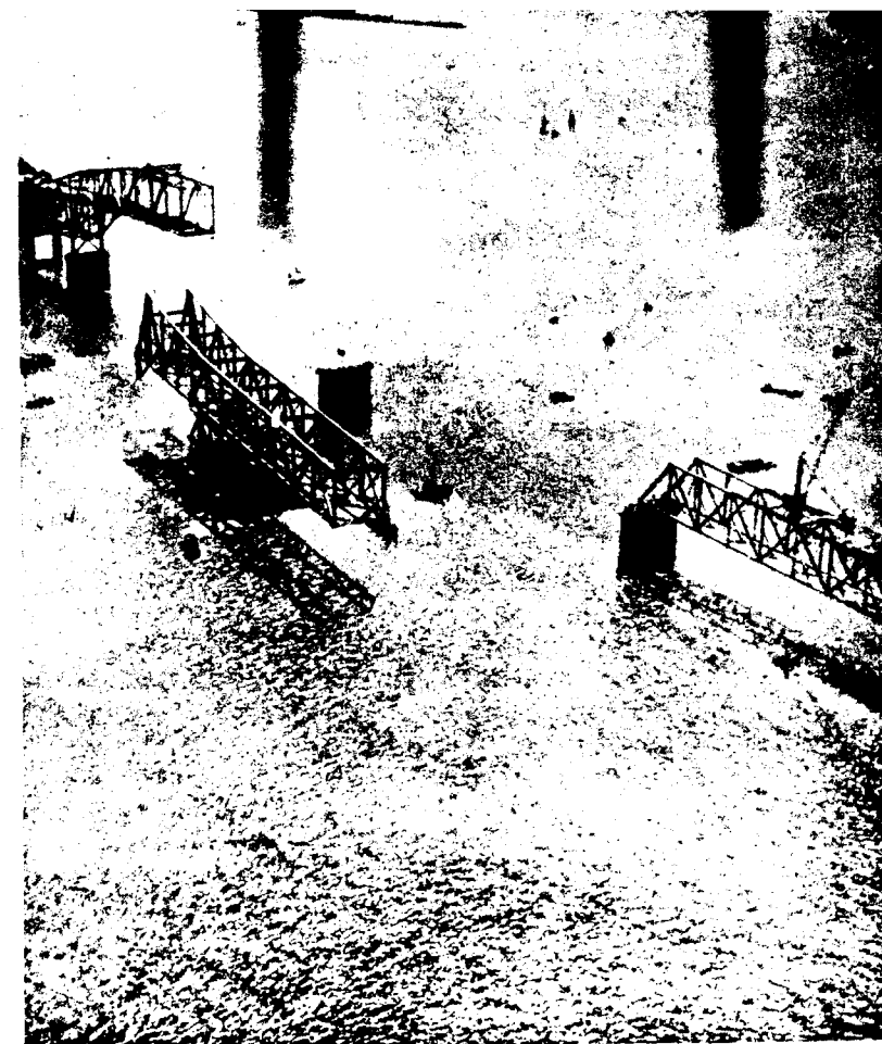
STAGES OF CONSTRUCTION. Tugs bring a unit of 1,200 tons of floating steel—built on a smaller span—into position for the final move, which took three and a half hours to complete. Right: an aerial view showing one of the floating middle sections and the gap it will occupy. Supported by 50,000 tons of concrete pier-work, buried in the rock bottom of the harbour, the bridge will carry 8,000 tons of roadway.
