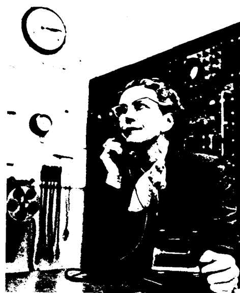
THE EXACT TIME is also given to Canadians over the telephone. The star observations determine the rates of quartz crystal clocks, used as primary standards.
