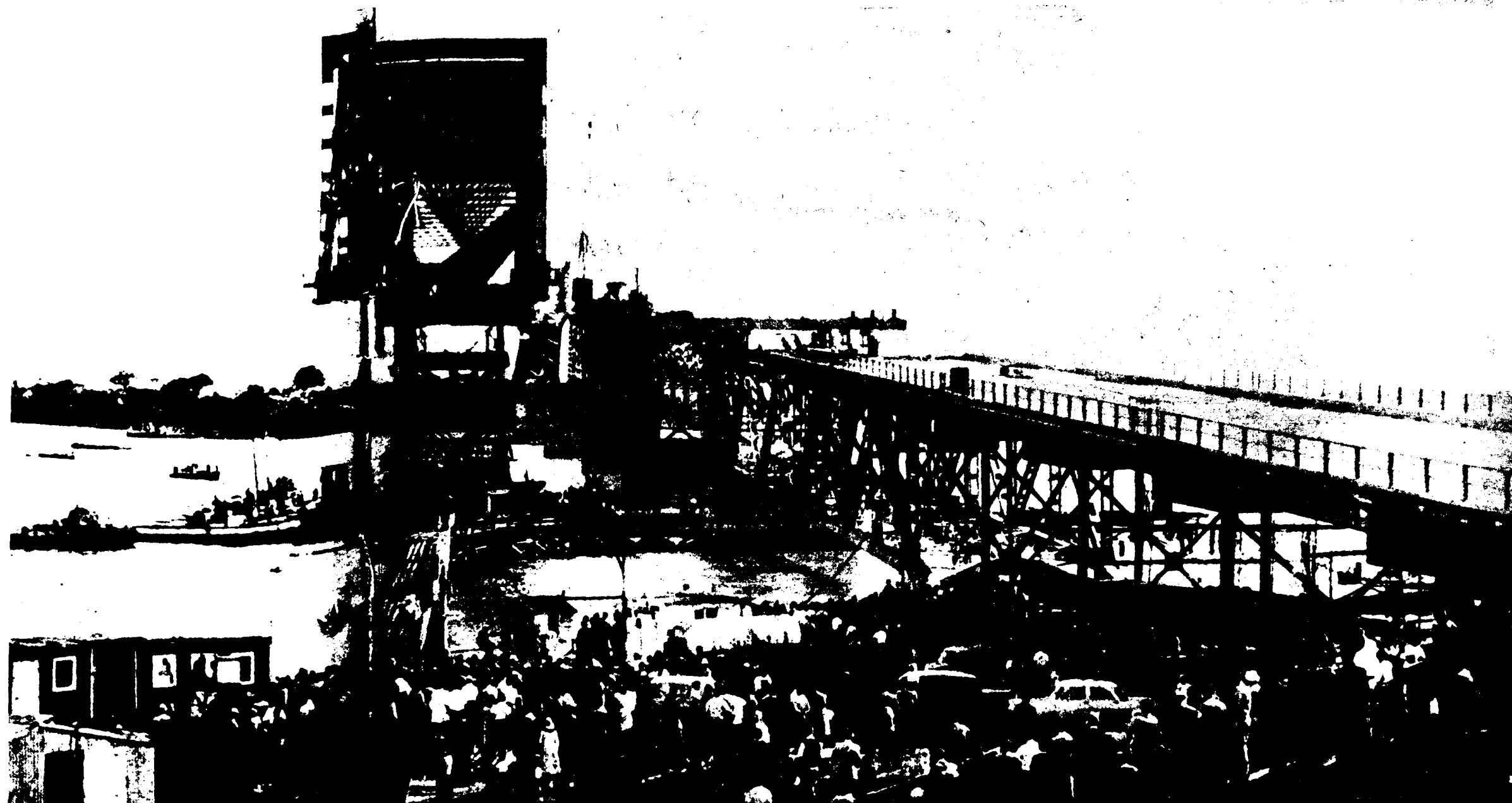
NEW ZEALANDERS watch as tugs and winches manoeuvre the "pick-a-back" middle section of the bridge out into the harbour. On the right of the picture is one end of the pier with its completed concrete roadway.
