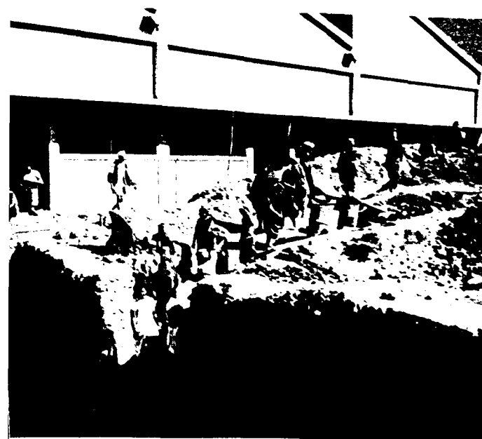
EXCAVATION work on a pit into which effluent storage tanks were installed. Waste liquids from the radiochemistry laboratory are collected in these tanks and later checked for radioactive contamination before being pumped into the sea.
