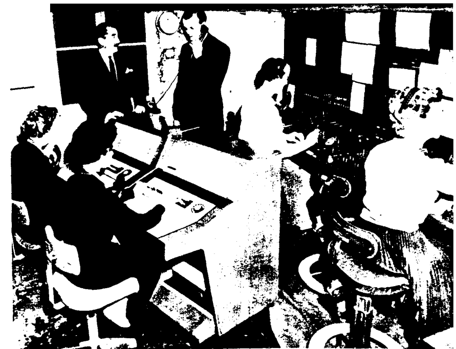
First Cordless Switchboard Goes into Action
