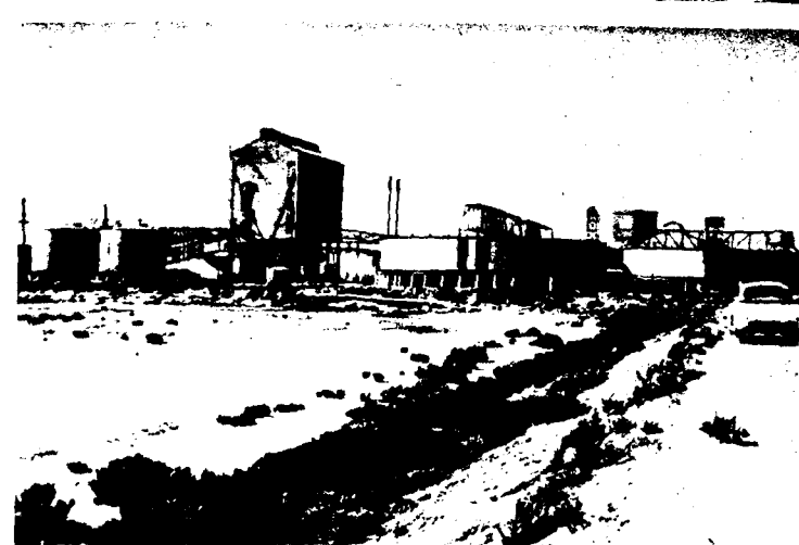
PORT PIRIE extraction plant, built on reclaimed land on Spencer Gulf by the South Australia Mines Department at a cost of £1,500,000. It operates throughout the week and has an annual output of 450,000 lb. of uranium oxide.
