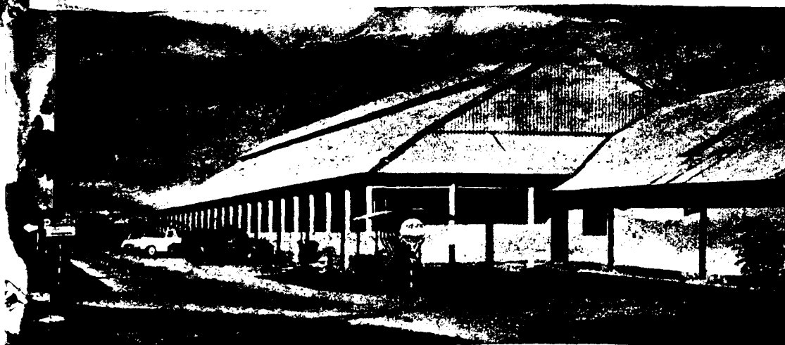
MINI-MARIAT building at Seria, Borneo, is an example of Situfoam used in conjunction with a reinforced concrete frame. Situfoam technique is well suited to tropical regions, where hundreds of such buildings have been built.
