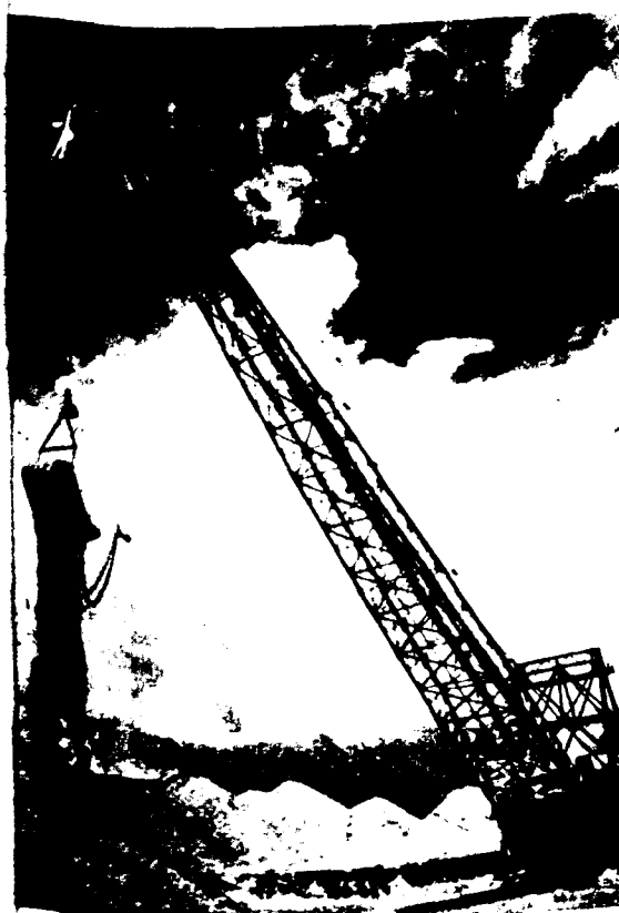
BAUXITE Walking dragline machine removing the sand and clay, sometimes as much as 50 ft. deep, covering the rich deposits of bauxite, from which aluminium is refined. This machine is one of the largest in the world. British Guiana exports some £5 million worth of this ore every year.
