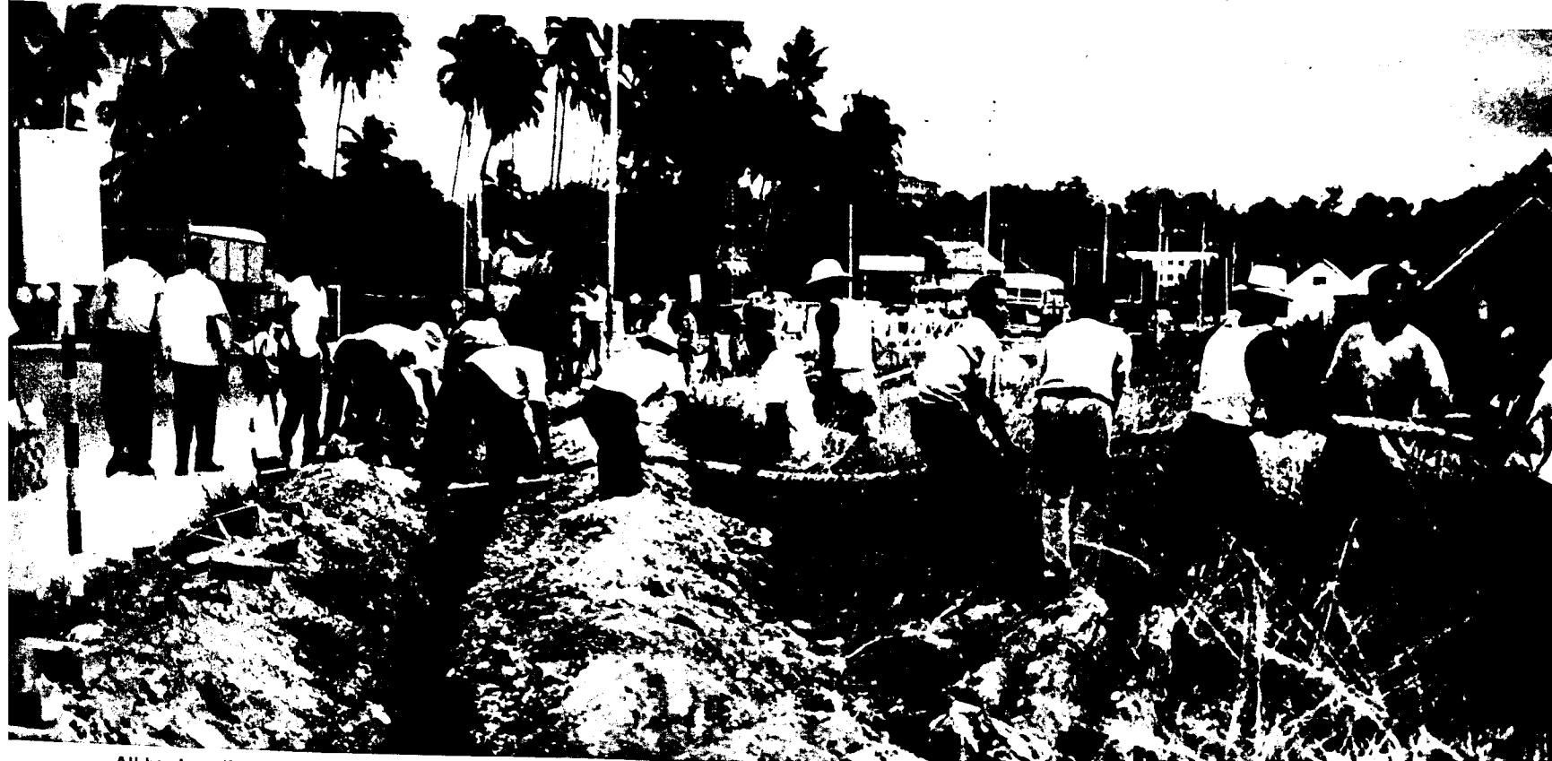
All hands on the job as a three-core 11 kV cable, manufactured by British Insulated Callender's Cables Ltd., is laid as part of a new ring main at Jesselton, Sabah. The cable was supplied for the Sabah Electricity Board, who carried out the installation
