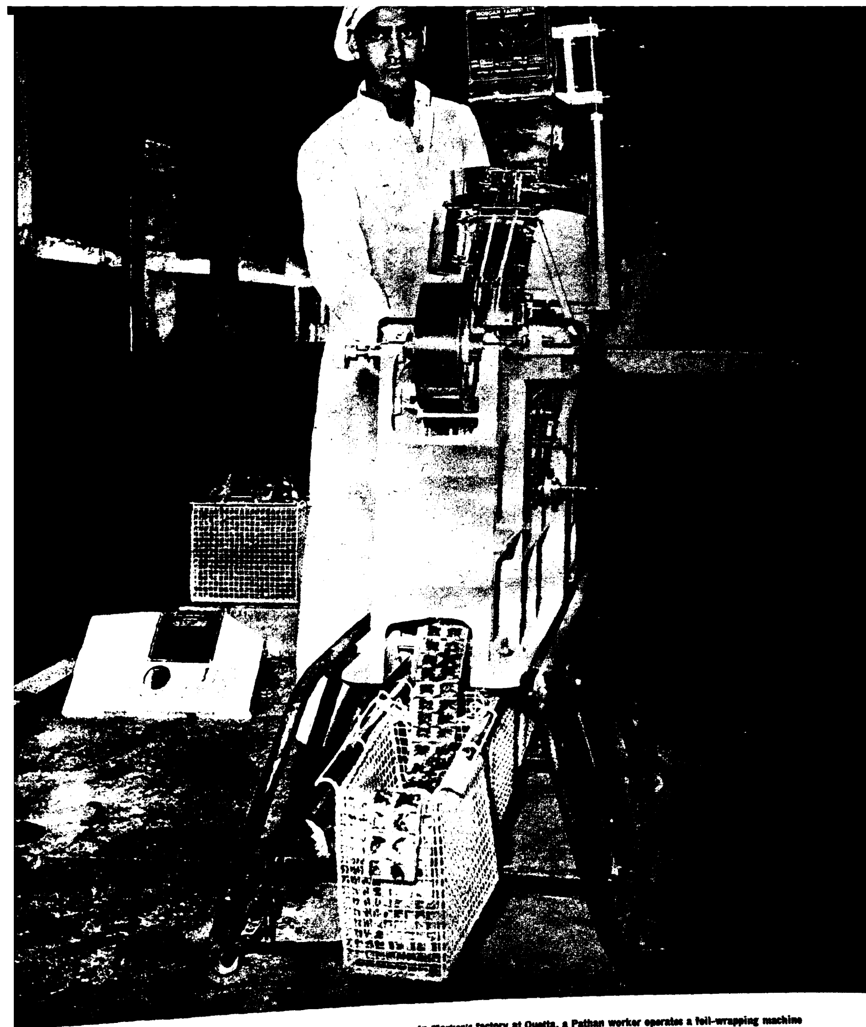
In Marker's factory at Quetta, a Pathan worker operates a foil-wrapping machine manufactured by Morgan Fairless Ltd., of Sheffield, England.
