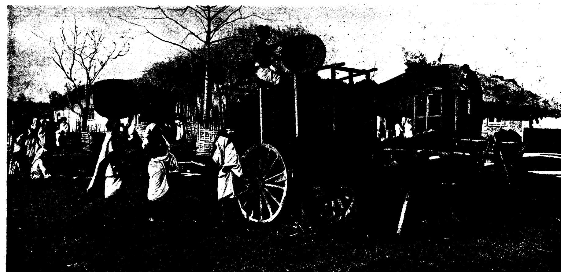
Tea leaf from an out-garden being loaded on to special chicken-wire buffalo carts for transport to the factory
