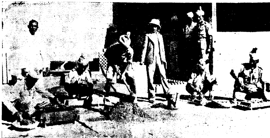
Soldiers being put through the cement course at the Baluch Regiment's training centre and (below) Some of the work completed by them.
