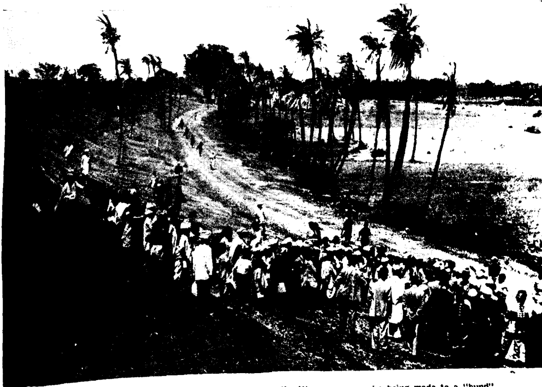
During his tour of scarcity areas in Mysore, the Viceroy saw repairs being made to a "bund" which forms part of the famine relief operations started by the Mysore State. Picture shows the villagers crowding round the Viceroy and the Maharaja of Mysore.
