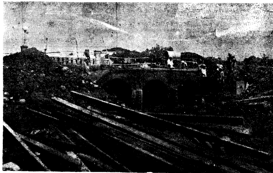
Note the Archway on the Downstream Side: Circular Openings are provided on the Upstream Side.
