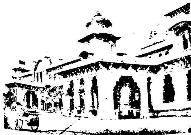
Egmore Railway Station
