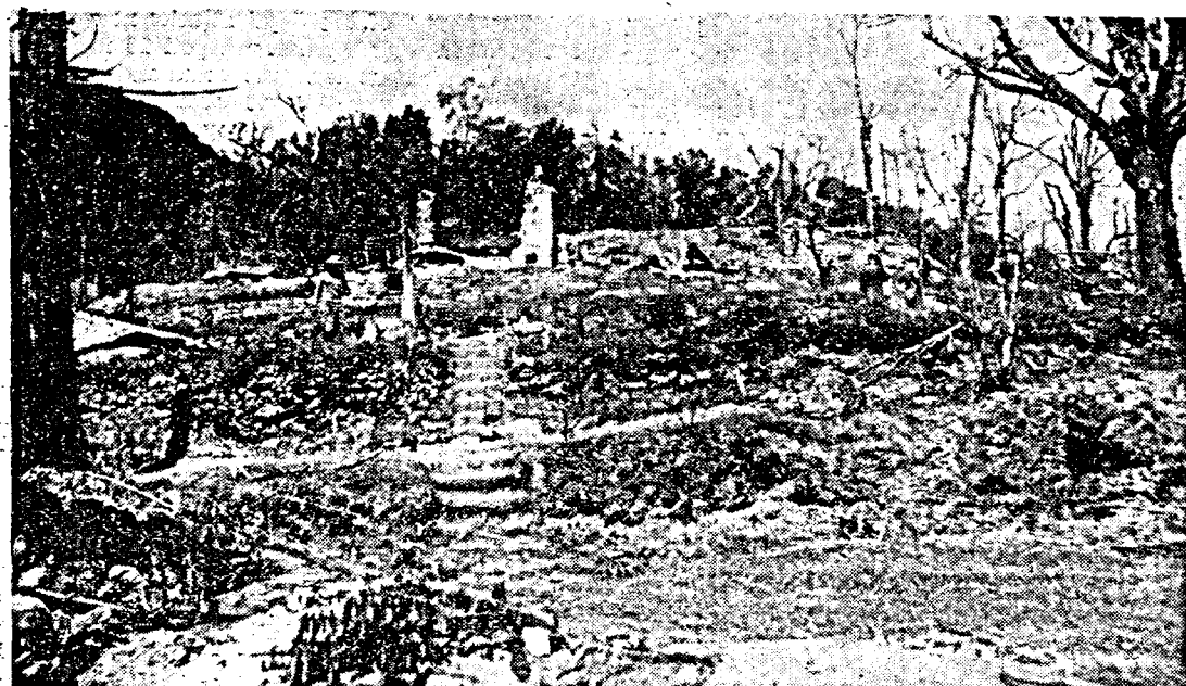
The ruined tennis court and terraces of the Deputy Commissioner's bungalow.
