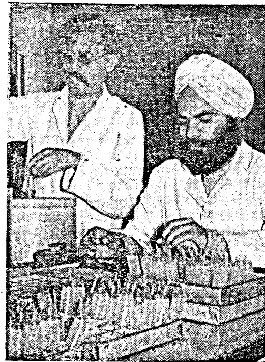
Sera and vaccines for Army and civilian use are produced at the Central Research Institute, Kasauli. Picture shows vaccine ampoules being sealed with a blow pipe.
