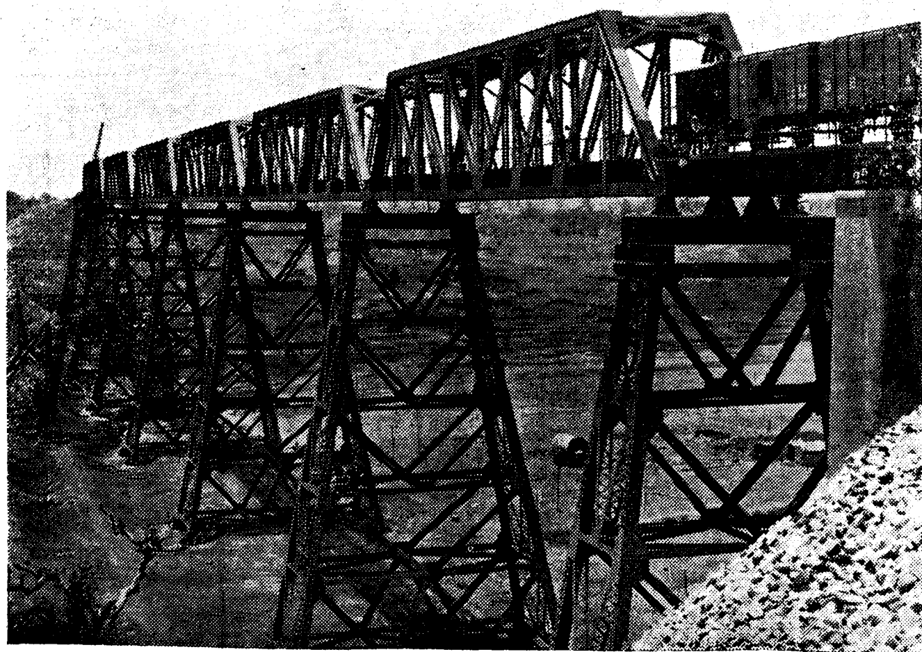
Nerbudda Bridge, G. I. P. Railway, 6 spans of 165-feet and 4 spans of 40-feet on 100-feet high Trestles.
