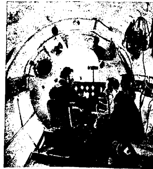
Pilots undergo pressure tests in this chamber and their response to orders given them through inter-communication telephone under these artificial conditions is recorded by various meters and gauges
