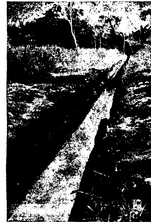
Stagnant water from a mosquito-breeding swamp in New Guinea is drained off through a canal dug by U. S. Army Engineers
