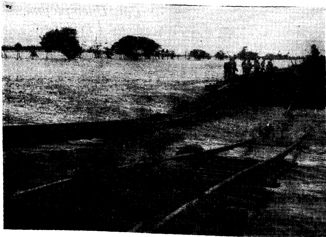
A breach in the double track to Calcutta.
