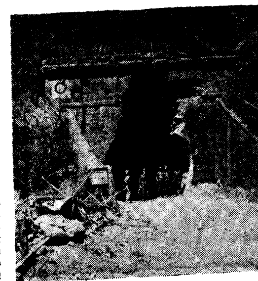
Shattered entrance to a tunnel on the Maungdaw-Buthidaung road, to which the Japs clung tenaciously.
