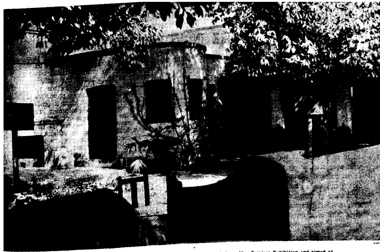
An exterior view of another Ideal Home built at the Lahore War Services Exhibition and aimed at the man with slightly larger means. This bungalow cost under Rs. 5,000.
