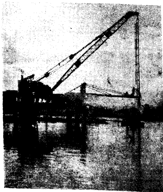
Piles being driven into the bed of the river for constructing a bridge.
