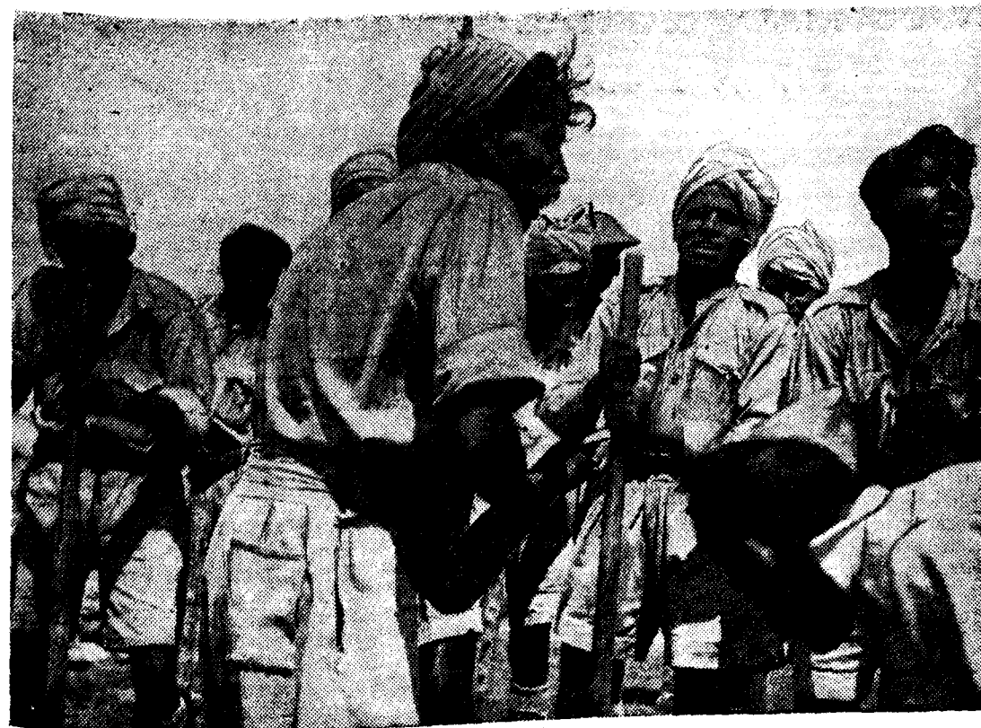
A Cochin State Labour Unit, engaged in military construction, work to "music", the man in the foreground beating a tin can.
