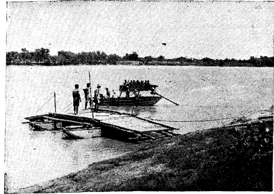
Rowing section of a pontoon bridge into position across a wide river.
