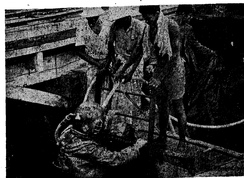
A Madras Sapper and Miner in a diving outfit: Ceylonese help him to climb in, adjusting his life-line and keeping a constant supply of air going.
