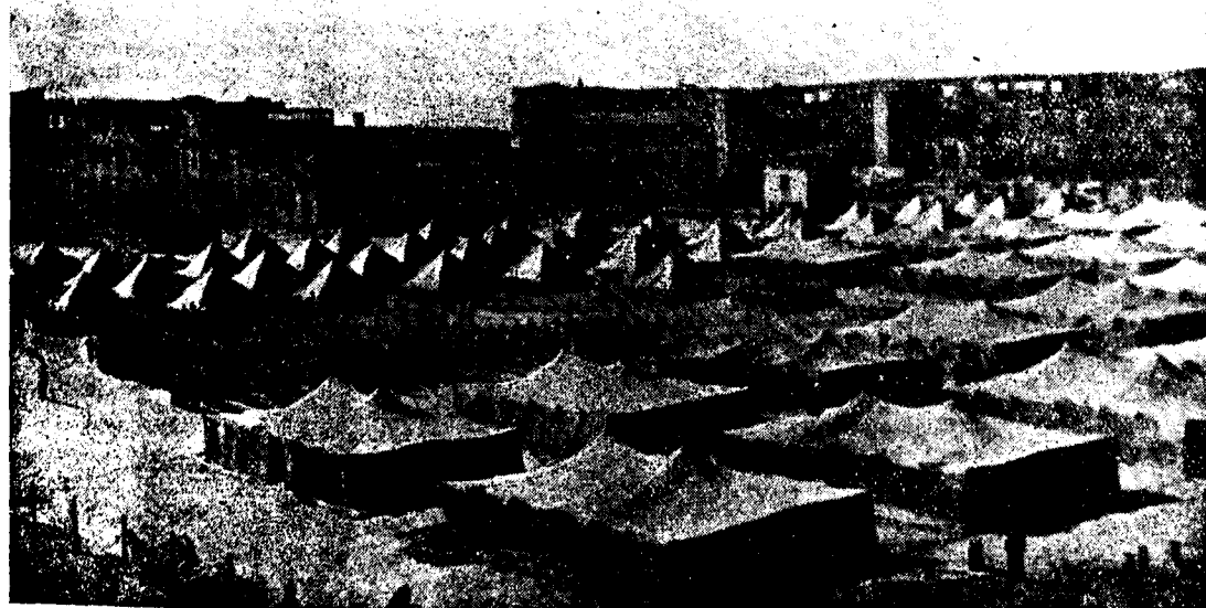
AFTER THE STALINGRAD VICTORY. —Heroic Stalingrad, demolished by Germans, is being restored. Photo shows Builders' Camp in one district of Stalingrad.
