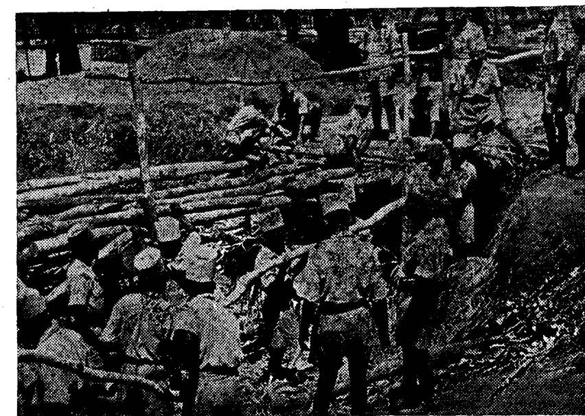
Madras Sappers and Miners bridge-building in Ceylon.
