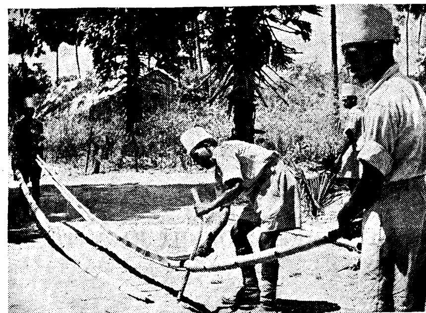
Splitting bamboos used in building huts in Ceylon.
