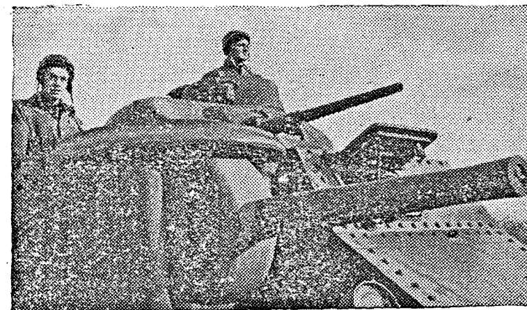
CANADIANS IN ENGLAND USE NEW SIX-GUN AMERICAN TANKS.—A Canadian Armoured Division training in Britain is now using new American-built "heavy-medium cruiser" tanks. Named after the American fighting Confederate leader "General Lee", these tanks each weigh 30 tons and carry one 3-inch gun and five machine guns. The massive armour-plating of this tank's superstructure is shown in this photograph of a "General Lee" manned by members of the Fort Garry Horse, a cavalry regiment famous in the last war.
