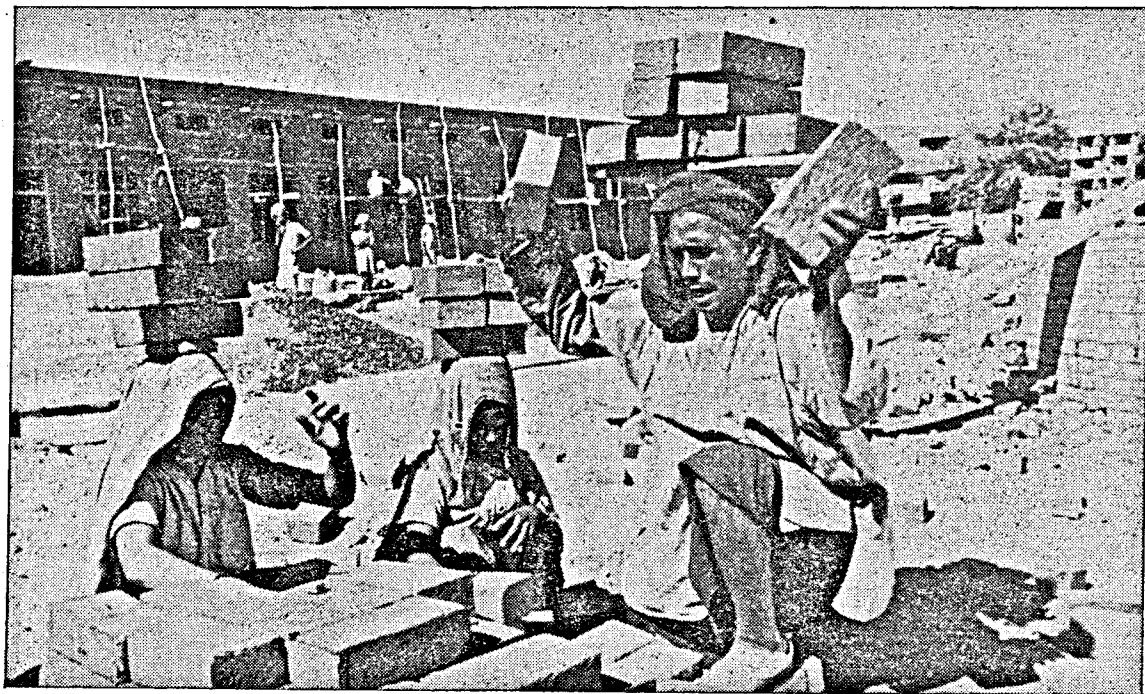
All over India, men and women are carrying and laying the bricks of new factories which are being built to produce various War supplies needed by Government. Photo shows part of a great quadrangular factory nearing completion.
