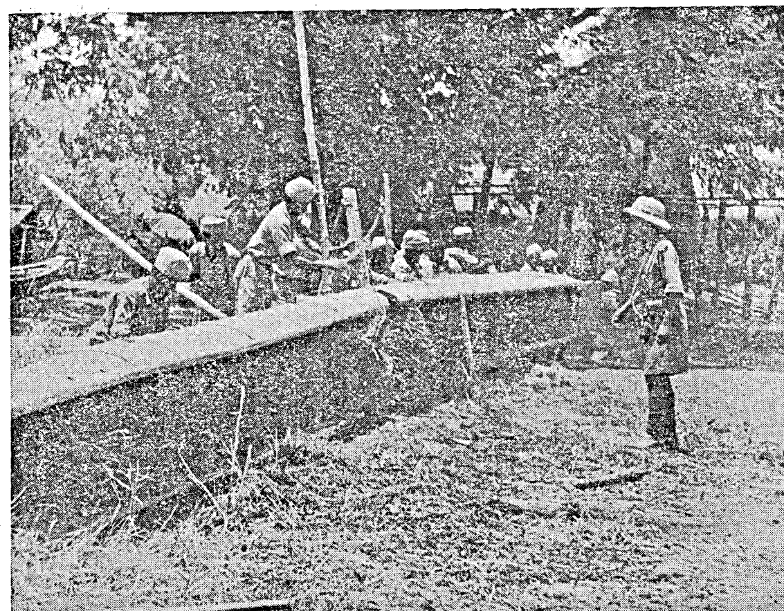
An Indian Labour Company near Ye-U at work on a boat which they are about to use for a pontoon bridge across a stream for our M. T. to cross.
