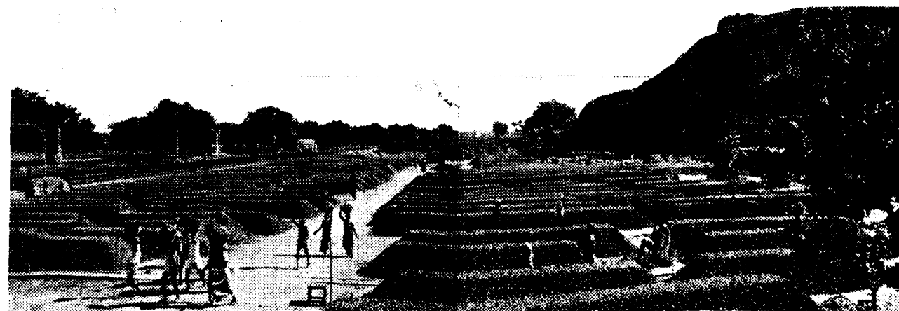
Known as 'Metal', whole mountains have been carved to provide stone 'ballast' for the Railway track.
