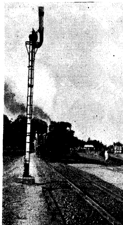
The New signal.
