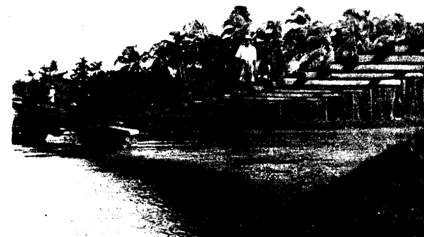
Breach spot near Pudukad on the Shoranur-Cochin Ry.
