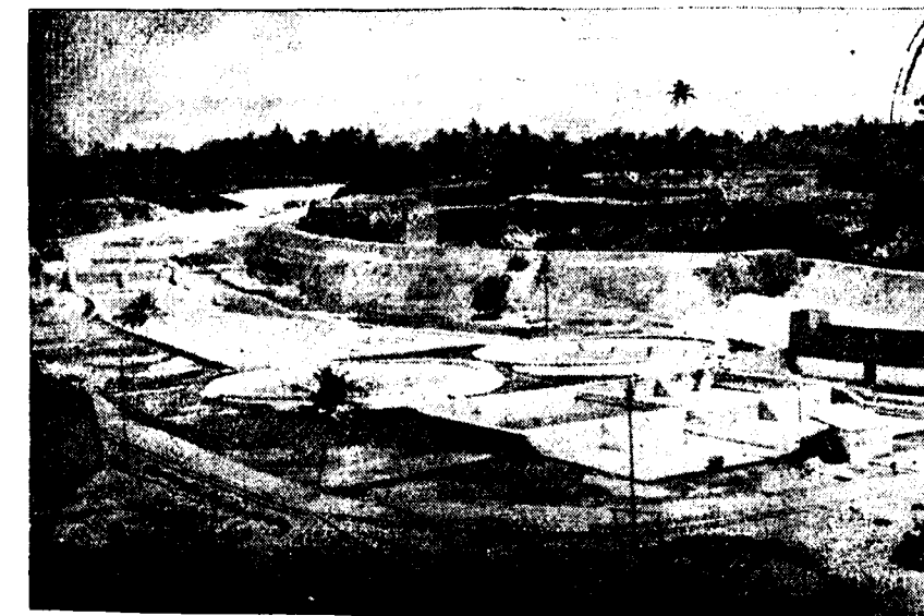
General view of the Clay Refining Plant.
