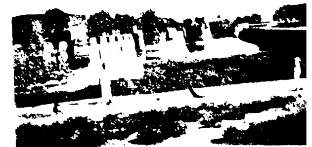
The Vellore Fort (T. R. Kothandaraman, II U. C.)
