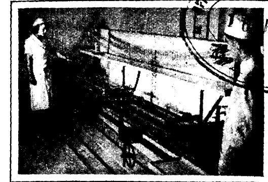
Precision Automatic Polishing, in one operation, of twelve catgut strands, each 10 feet in length.
