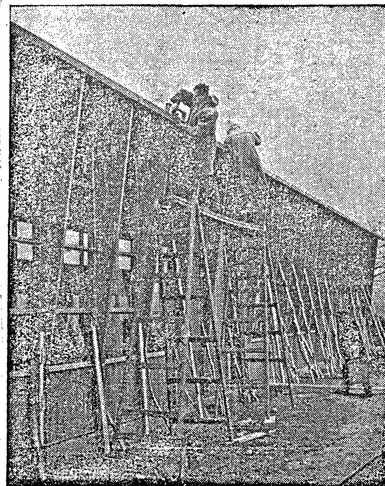
The first of several to be erected in Britain, an aluminium school, the New Mundella County Primary School, is being built at Park Farm Road, Folkestone, Kent. Others are to be erected at Maidstone, Sidcup, Erith and Dartford. In this picture, workmen are seen fixing gutterings to one of the classroom blocks.
