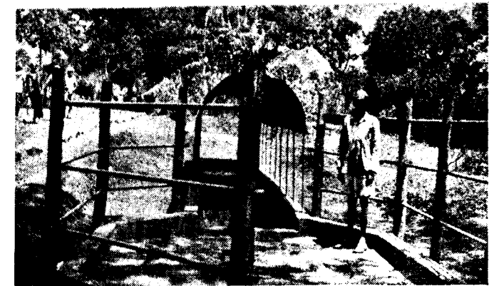
Fig. 2. Photo of the Cattle Dipping Tank at Turkewadi, Belgaum Dt. (Front View)
