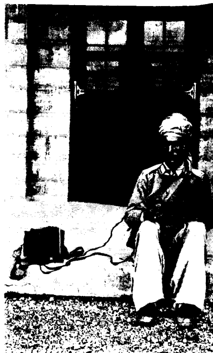
Shoulder harness slipped off and the set in use with quarter wave aerial on the ground. Switch and tuning dial just visible on top of the instrument case
