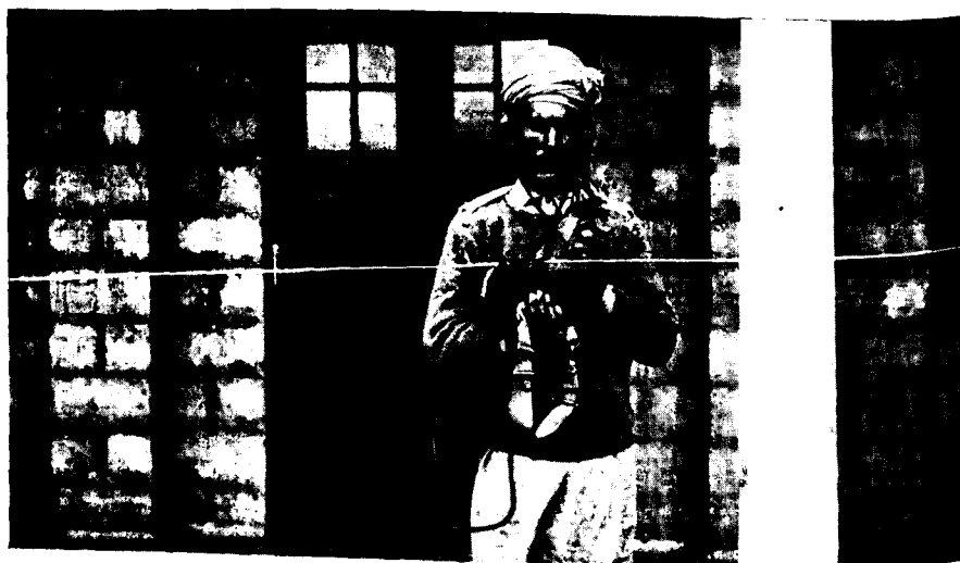
Set in use with the dipole aerial. It can be held and operated thus very simply, otherwise put on rocks, walls, etc.
