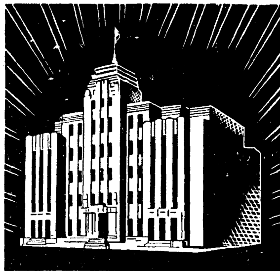
Head Office Building, Madras. Under Construction.
