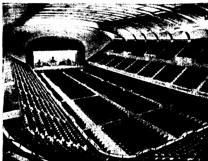
CLEVELAND PUBLIC AUDITORIUM—ARENA WITH SEATS IN PLACE
