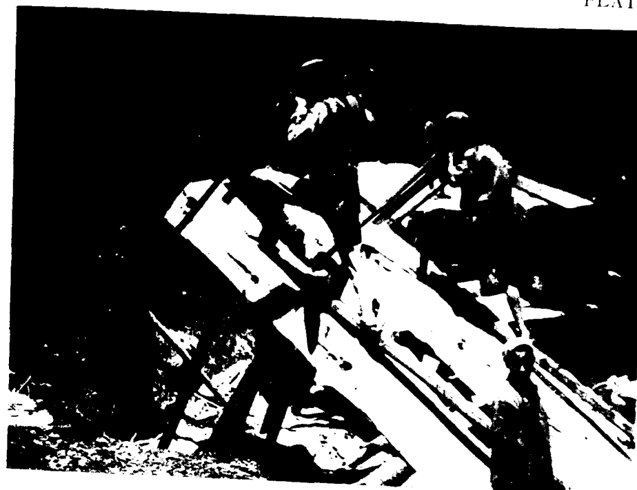
SAWING PAIRS MAKING DEODAR SLEEPERS.
