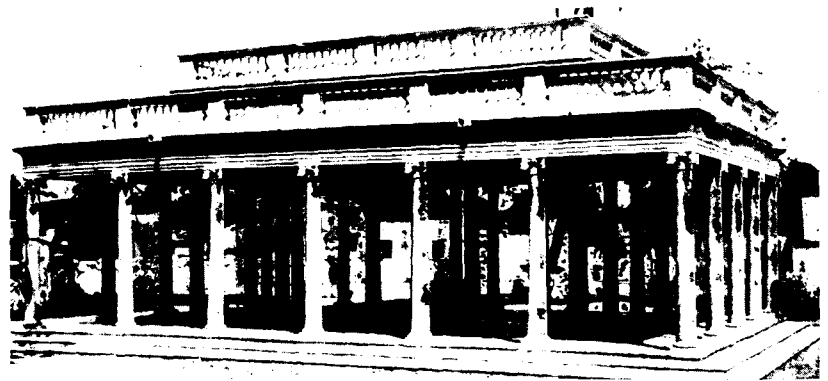
PAVILION IN CHILDREN'S PARK, HYDERABAD.
