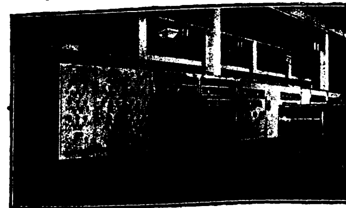
One of the 50-kW TRANSMITTERS that have been installed at the Empire Station at Daventry, showing (left) the crystal oscillator and frequency-doubling stages, and (centre) the intermediate amplifying stages and output stage. The modulator stages are on the right. (By courtesy B.B.C.)
