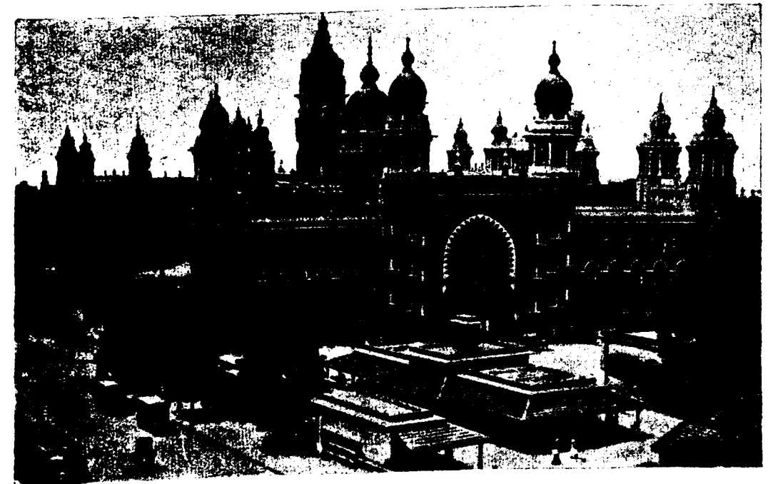
THE HIGH COURT BUILDINGS, MADRAS.
