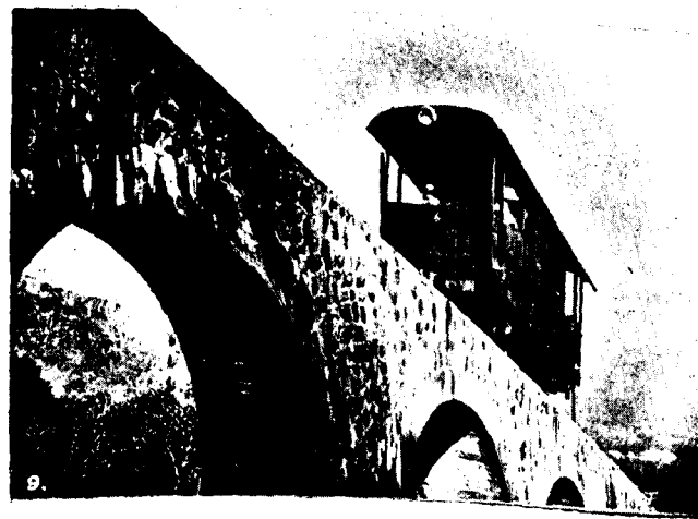
PENANG HILL RAILWAY: A detail from a Bridge.
