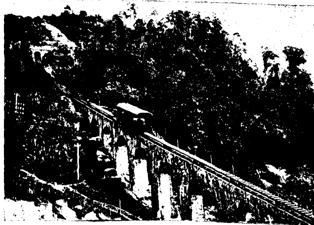
PENANG HILL RAILWAY: The Entrance of the Tunnel.
