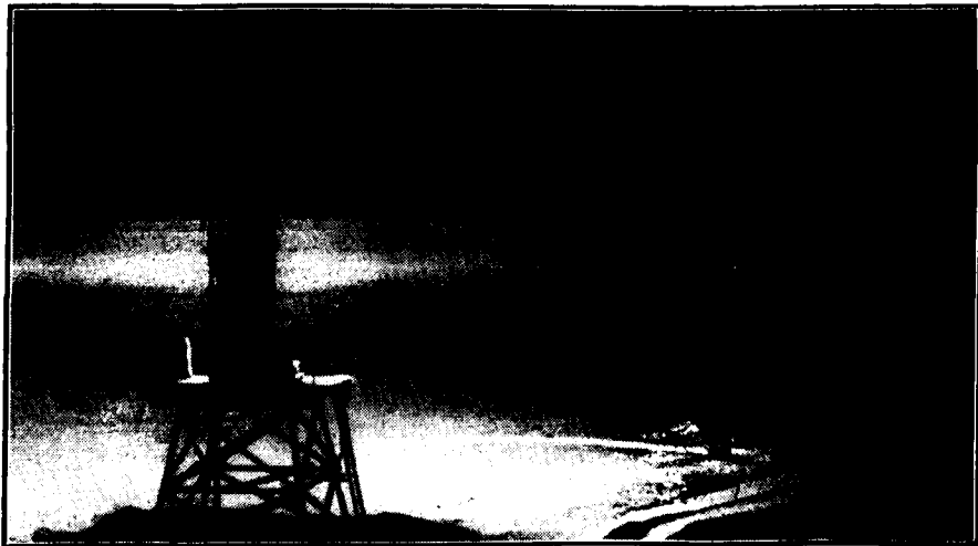
G. E. C. 9 kw. shadowbar landing floodlight beacon, Dum Dum Aerodrome.
