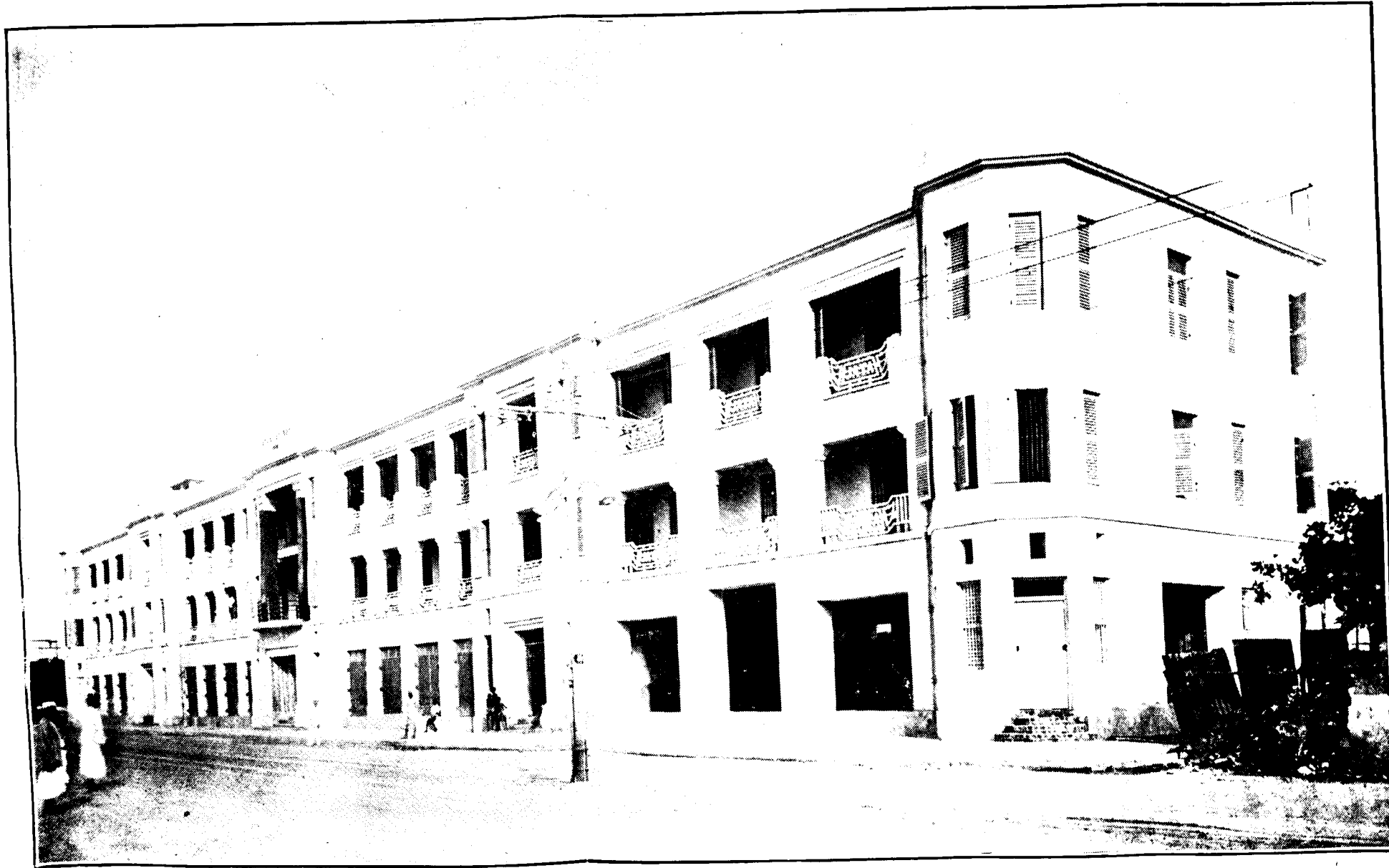
JAYA MANSION, FRONT VIEW.
