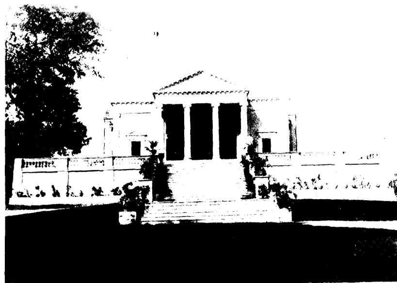
GUEST HOUSE, BASHIR BAGH, AFTER IMPROVEMENT.
