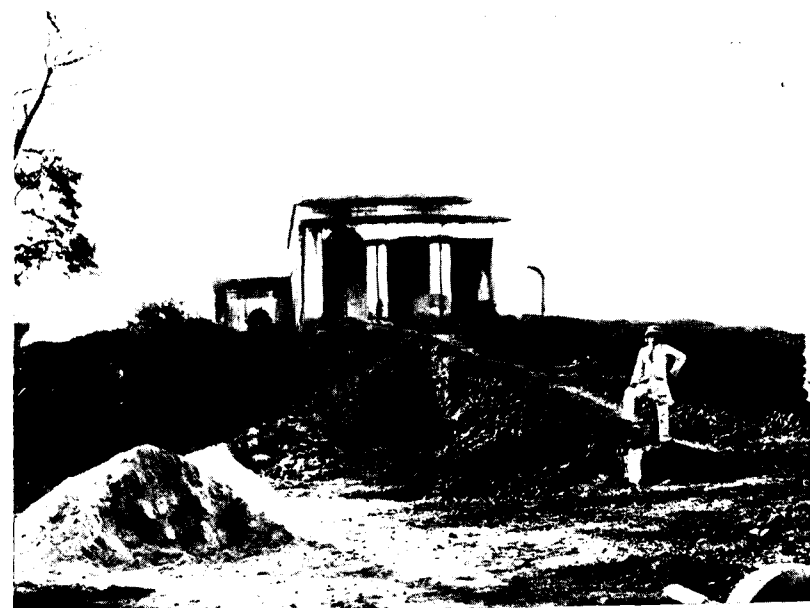
GUEST HOUSE, BASHIR BAGH, BEFORE IMPROVEMENT.
