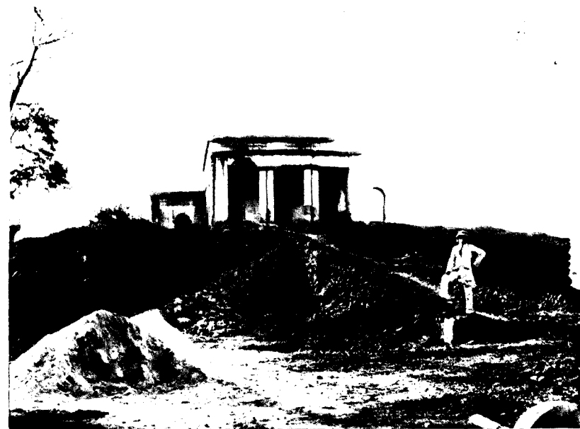
GUEST HOUSE, BASHIR BAGH, BEFORE IMPROVEMENT.
