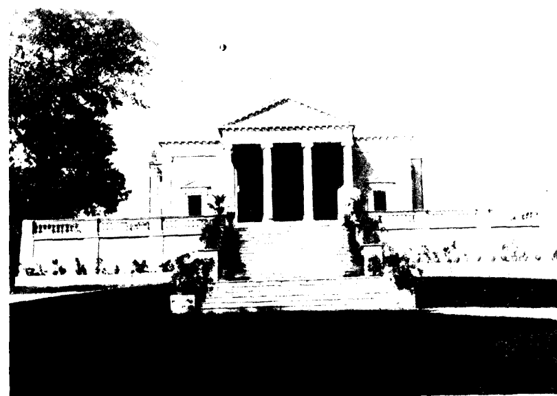
GUEST HOUSE, BASHIR BAGH, AFTER IMPROVEMENT.
