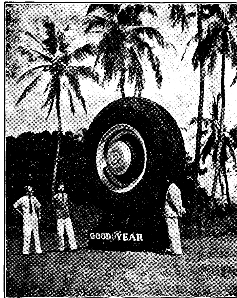
This concrete tyre, which has been recently erected at Worli, Bombay, is a landmark to motorists coming into and leaving Bombay. It was designed to the order of The Goodyear Tyre & Rubber Co. (India), Ltd., by their Advertising Agents Messrs. L. A. Stronach & Co. (India), Ltd., and was built and erected by The Simplex Concrete Works of Bombay.
