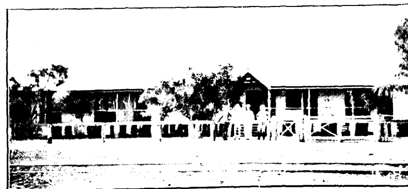
DERBY POLICE STATION AND QUARTERS
