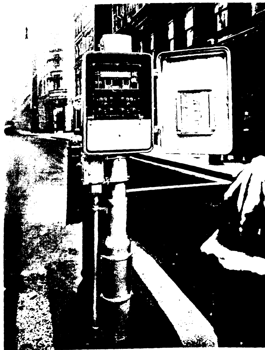
ELECTRO-MATIC CONTROLLER AT THE CORNHILL BY BISHOPSGATE, CITY OF LONDON, INTERSECTION (THE DOOR IS OPEN, SHOWING CONTROL SWITCHES)
