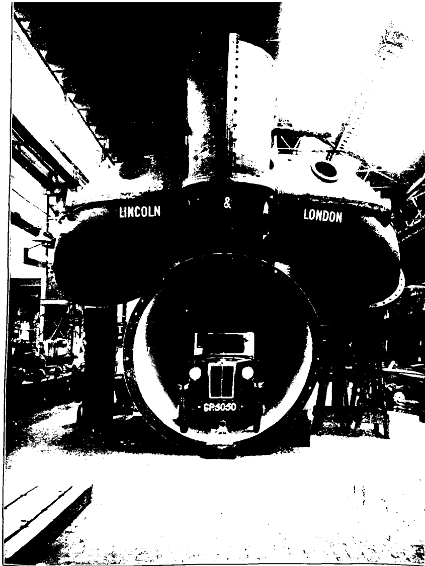
FIG. 4.—One of the three pumps of the new sluice.
