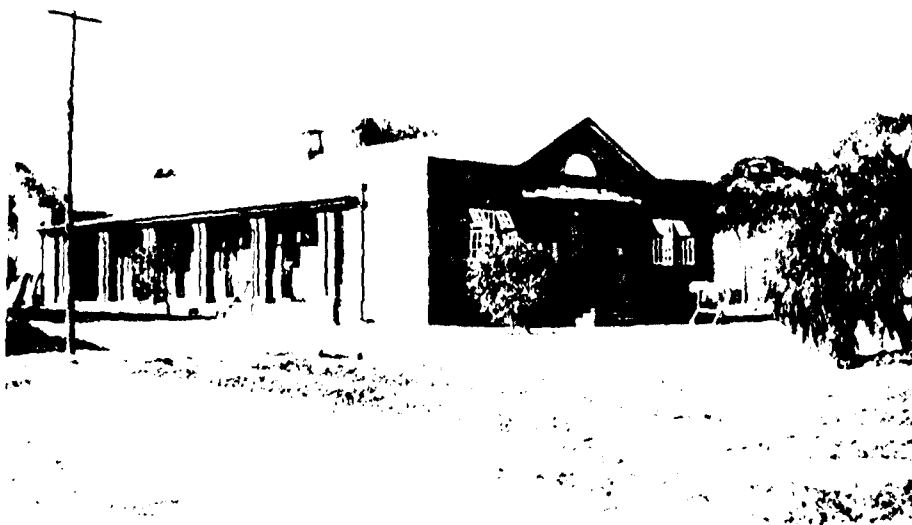
BARRACK ROOMS, HEADQUARTERS, SALISBURY BRITISH SOUTH AFRICA POLICE
