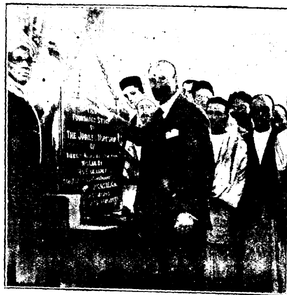
H. E. The Governor laying the Foundation-stone for the Silver Jubilee Workshop.
