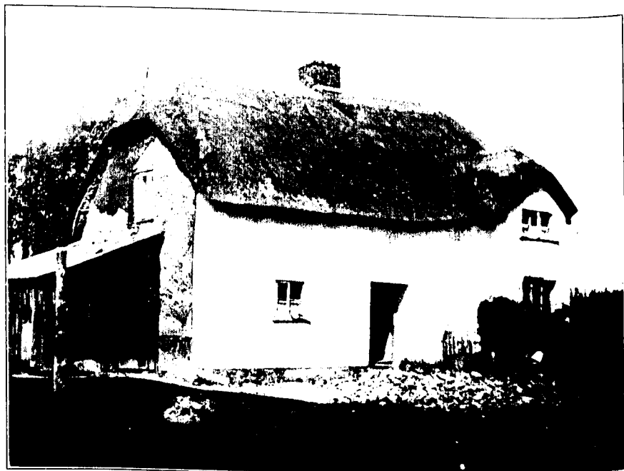
FIG. 4. Cottage (possessing archaeological interest) before reconditioning. The owner desired to remove the bay and thatched roof, but has been requested to submit revised scheme so that these picturesque features may be retained.
