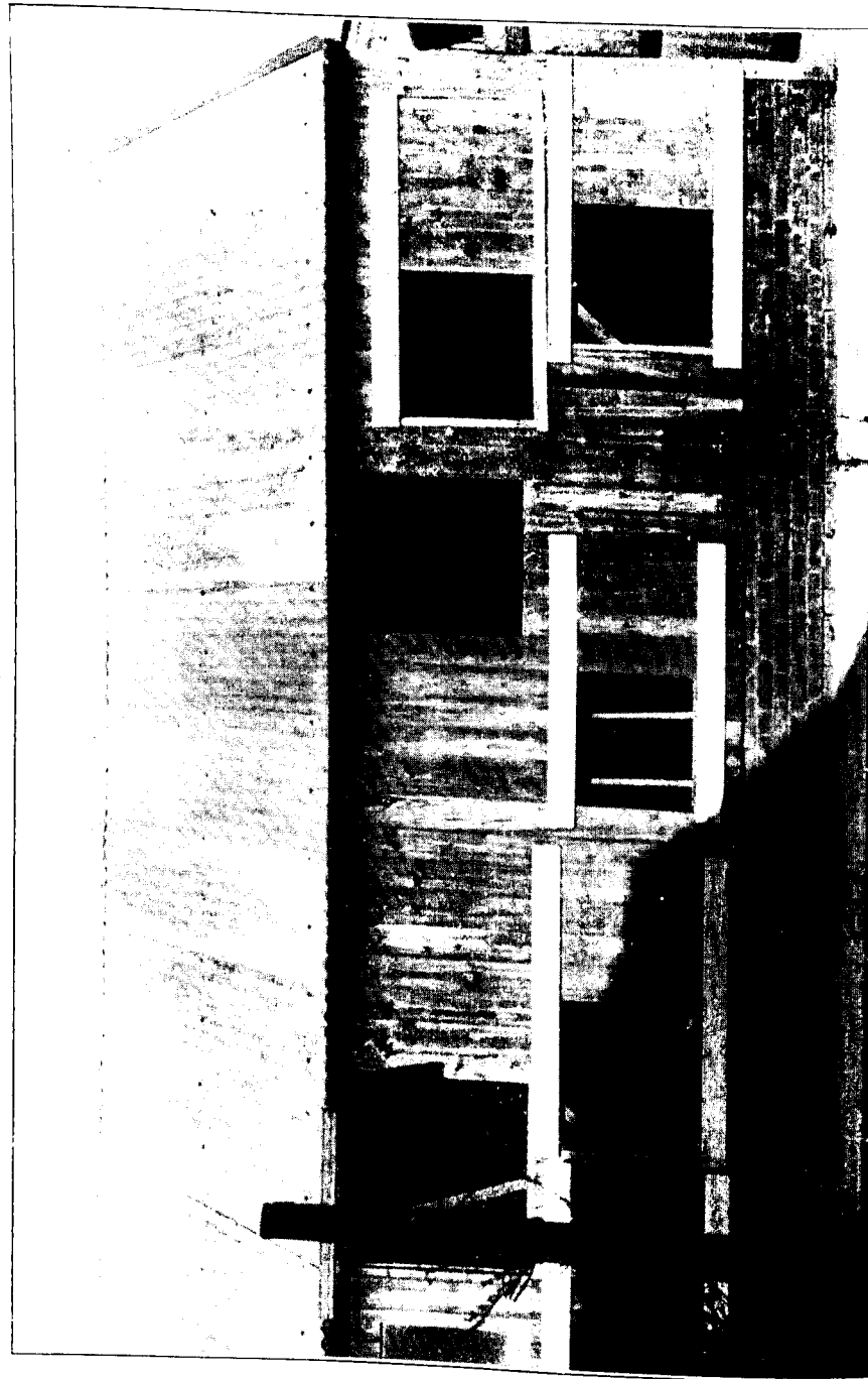
Fruit store successfully converted into a brooder house by introduction of openings into the south-east wall.
