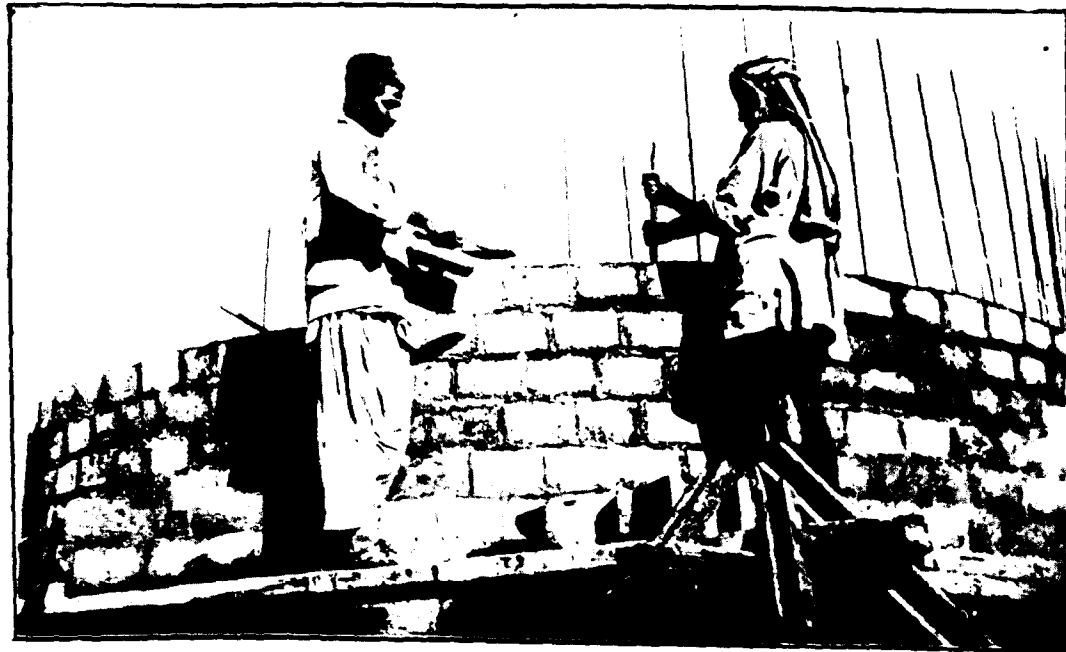
FIG. 1. Circular water tank under construction. The wall is nine inches thick.
