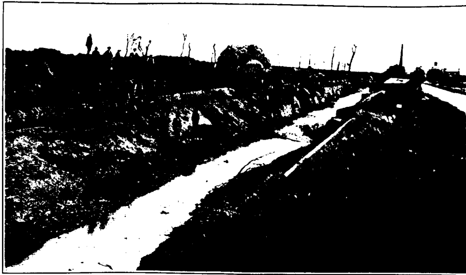
FIG. 7.—Sinking and Widening the White House Drain—lower end.
