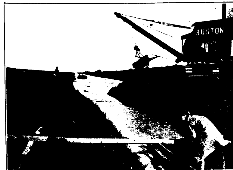
FIG. 5.—Drag-line Dredger at work.
