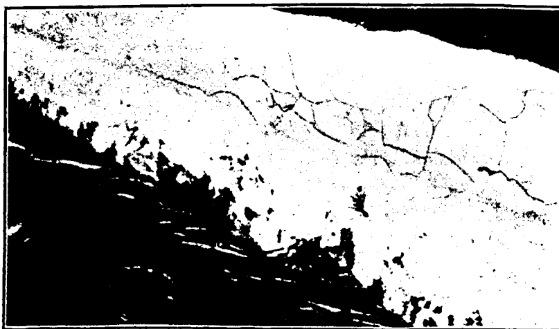
FIG. 4. Chicken wire and concrete plaster lining damaged by erosion and temperature cracks.
