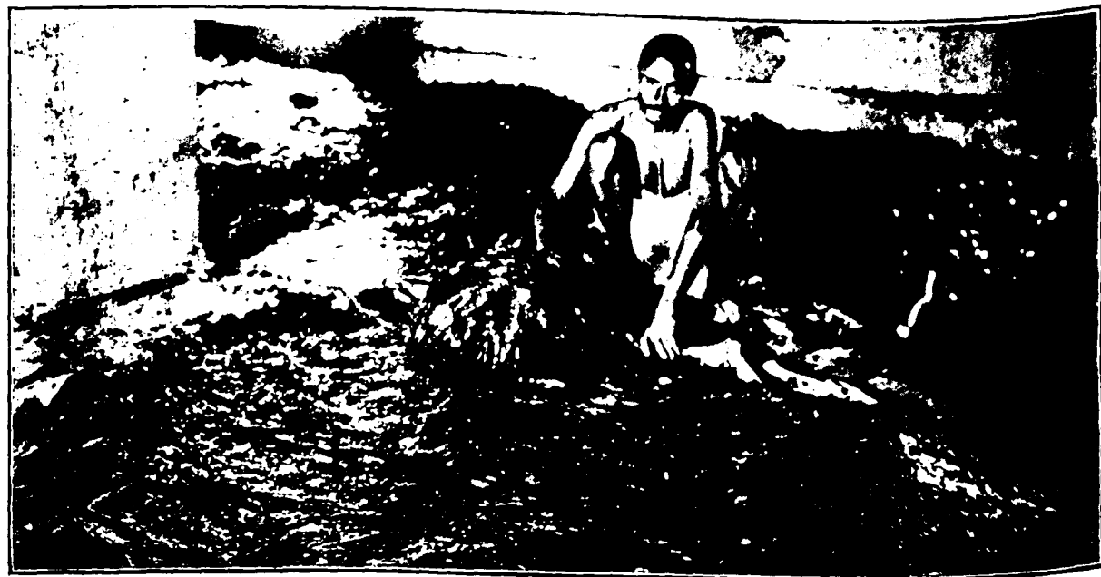
B. Aerating shellac during the hot weather. (Original.)
