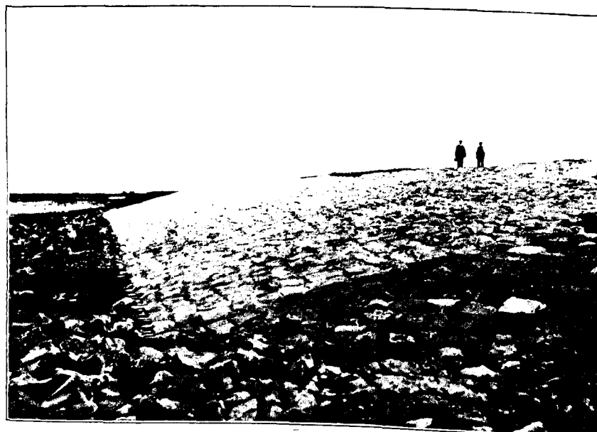
FIG. 10. Wick Sea-bank, Clevedon, Somersetshire: Showing portion of Bank re-inforced with stone pitching.
