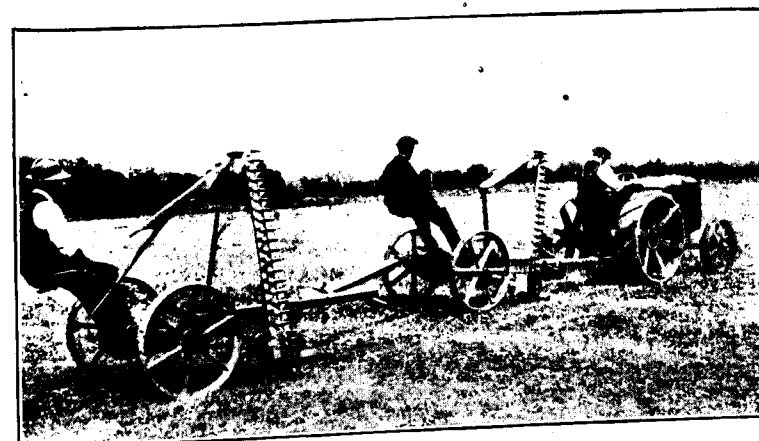
FIG. 1.—Two Bentall Mowers coupled by Kingdon Hitch.
