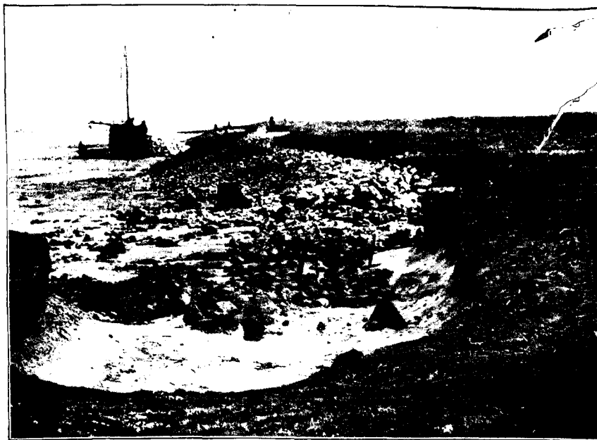
FIG. 9.—Wick Sea-bank, Clevedon, Somersetshire: Showing undermining of Bank by Tidal Scour.
