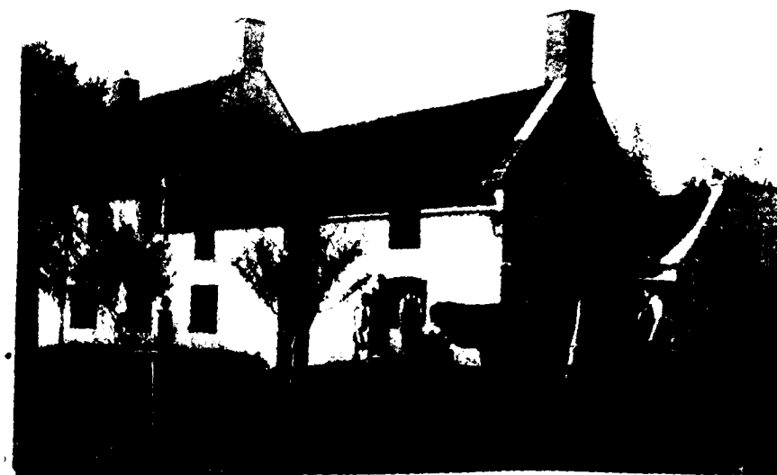
FIG. 2.—The same building as a Farm School.
