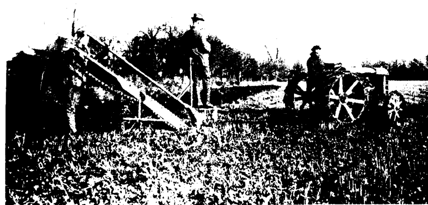
FIG. 6.—Swedish Excavator and Fordson Tractor.
