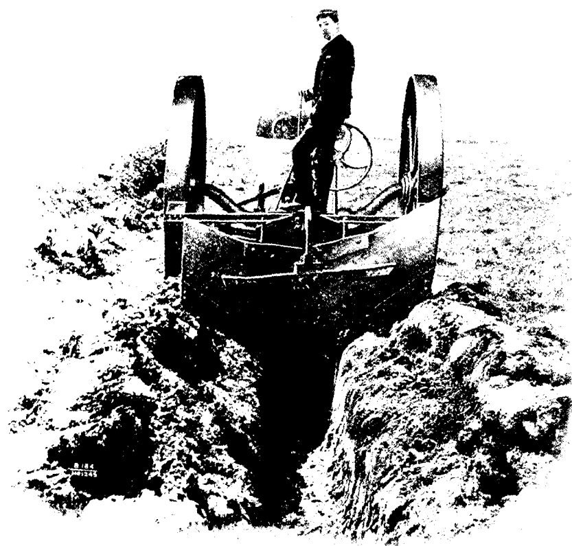
FIG. 12.—Fowler Trenching Machine at Work.
