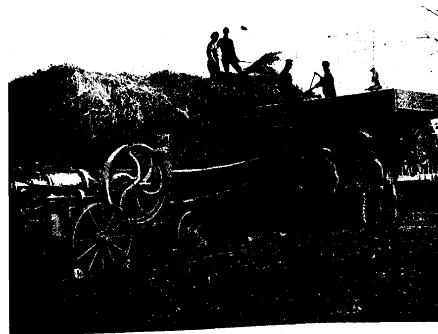
FIG 2.—6 to 8 B.H.P. Portable Oil Engine driving medium-size Thresher.
