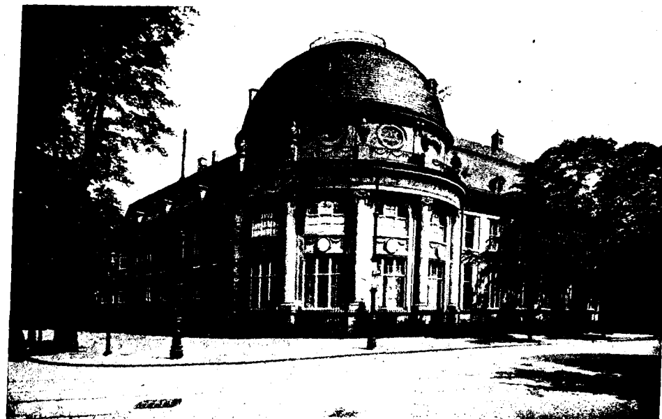
FIG. 5.—State Institute for Applied Botany and Seed Control Station, Hamburg, from Jungiusstrasse.
